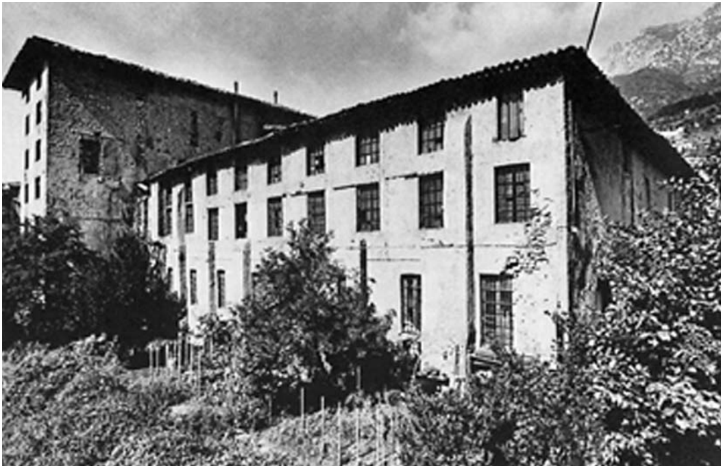
The Bovara spinning mill at Parè, seen from the south.
